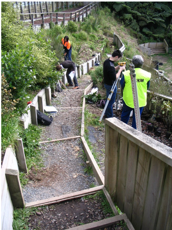
Geotechnical Engineer, Karen Jones, overseeing graduates undertaking soil and topographical survey for the Waharoa.
